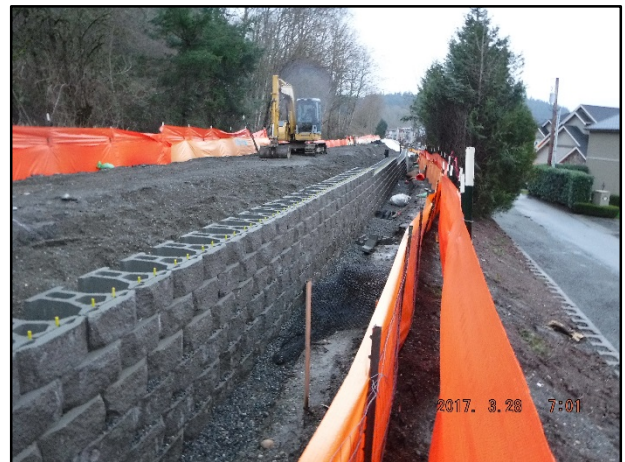
Continued block installation at Wall #6
