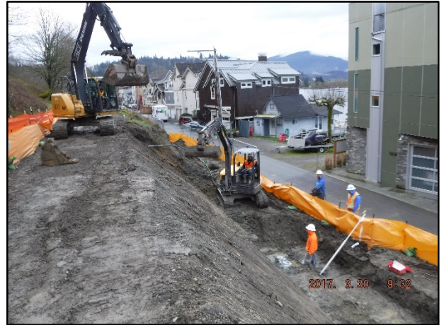
Continued excavation at Wall 4 and 5
