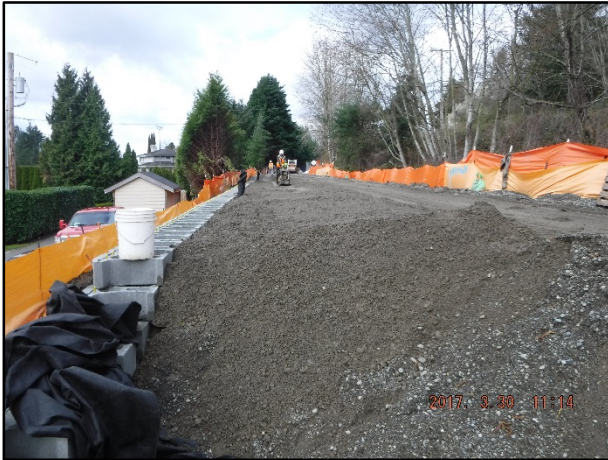
Continued installation of backfill at Wall 6
