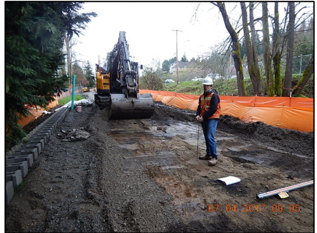
Excavation for trail asphalt base installation (CSBC)
