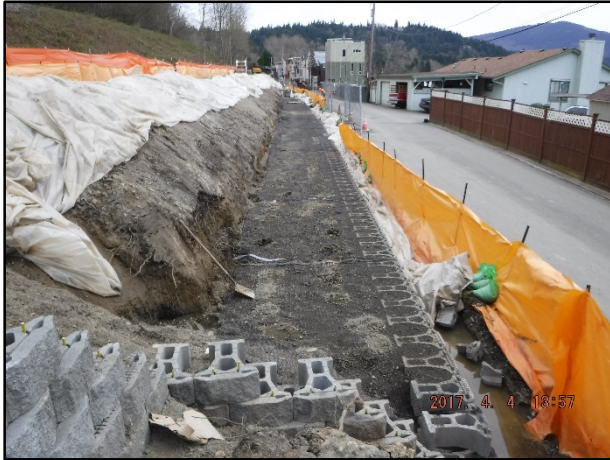
Continued construction of wall 5 and wall 5a
