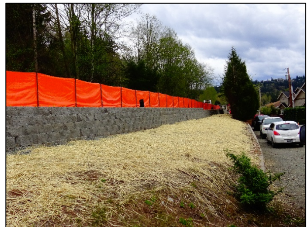
Safety fencing installed above completed portion of Wall 6
