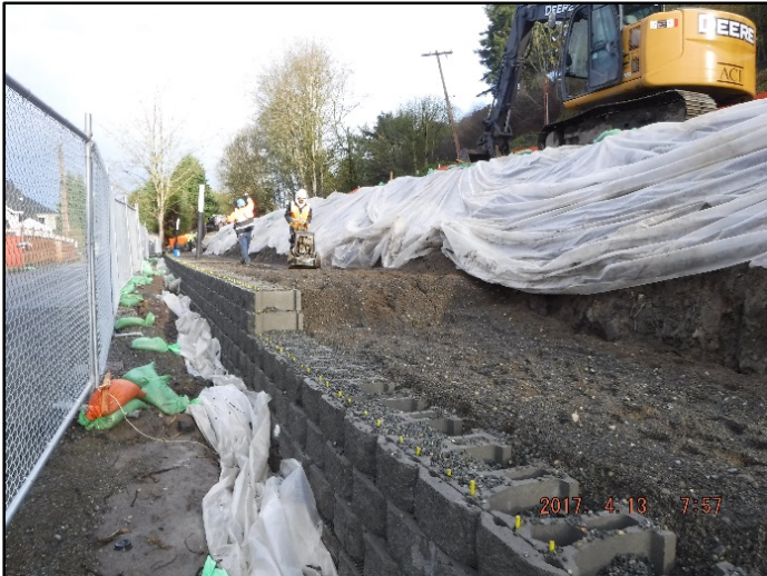
Continued backfill placement and compaction application at Wall 5
