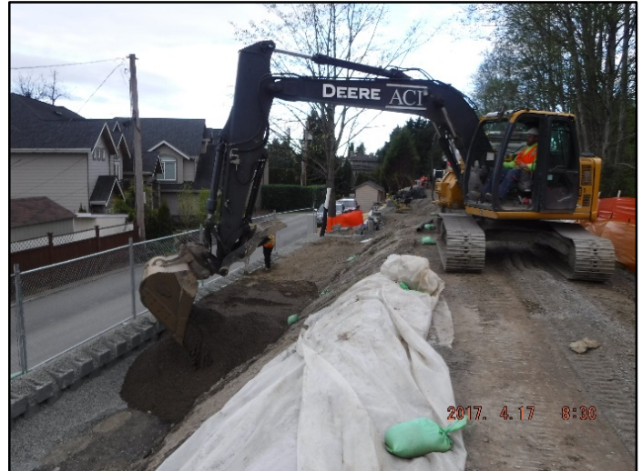
An excavator places backfill material at Wall 5
