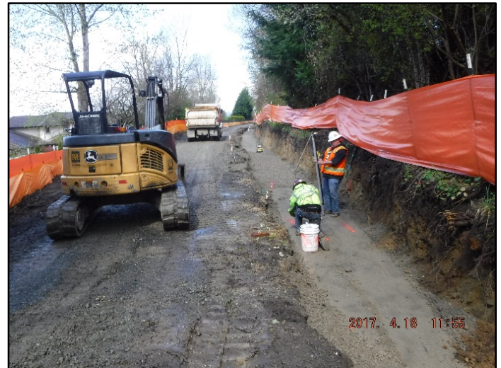
The contractor continues to construct Wall 8a
