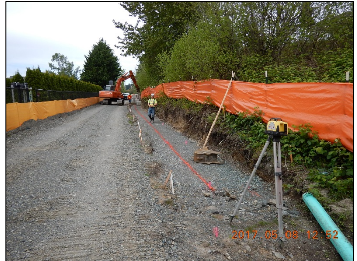
The contractor beginning installation of gravity block wall 8
