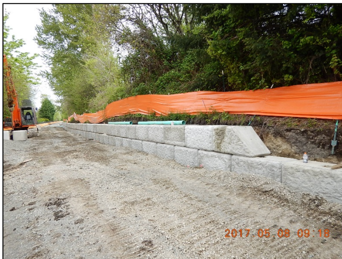
Continued block installation at gravity block wall 8 and wall 8a
