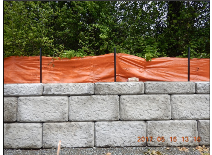
Chain link fence post installation above gravity block wall #8
