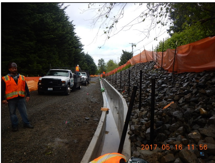
Chain link fence post installation behind the concrete channel
