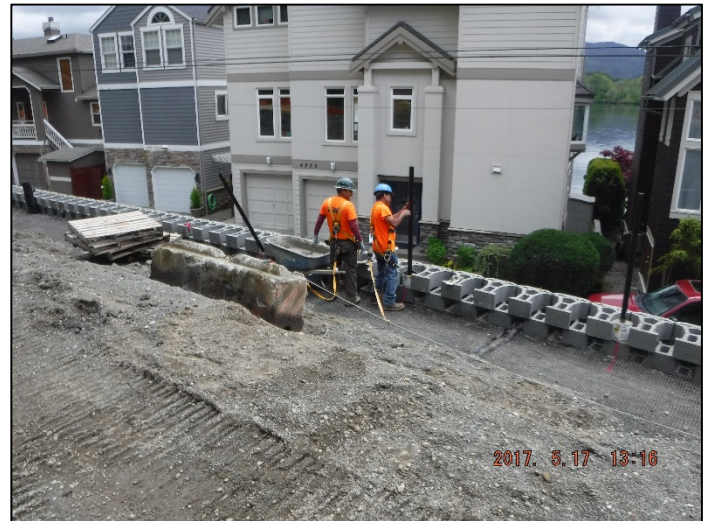
Workers safely installing chain link fence post installation within SEW Wall #5.
