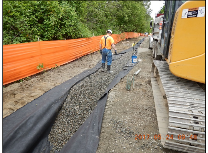
Infiltration trench installation
