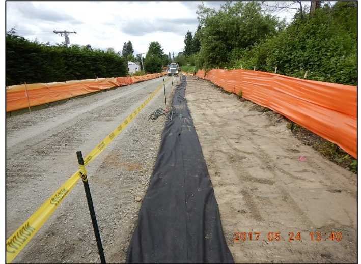
Infiltration trench installation between driveway 6 and 7
