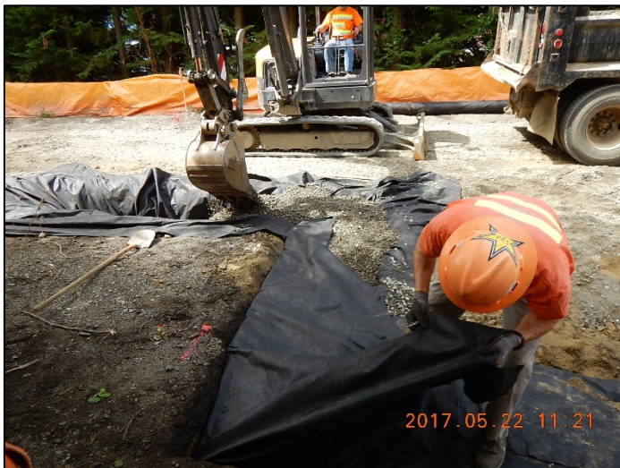
Infiltration trench installation near rest stop at 250+50
