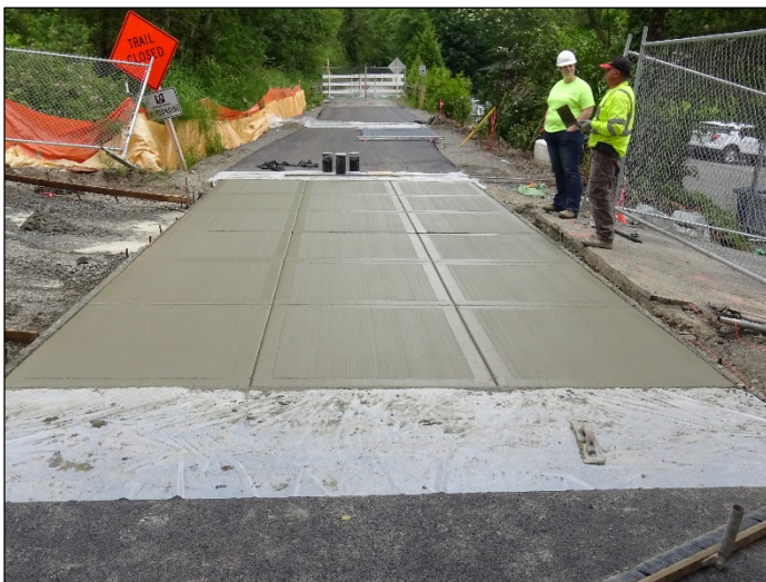
Completed, patterned trail intersection at driveway #1.
