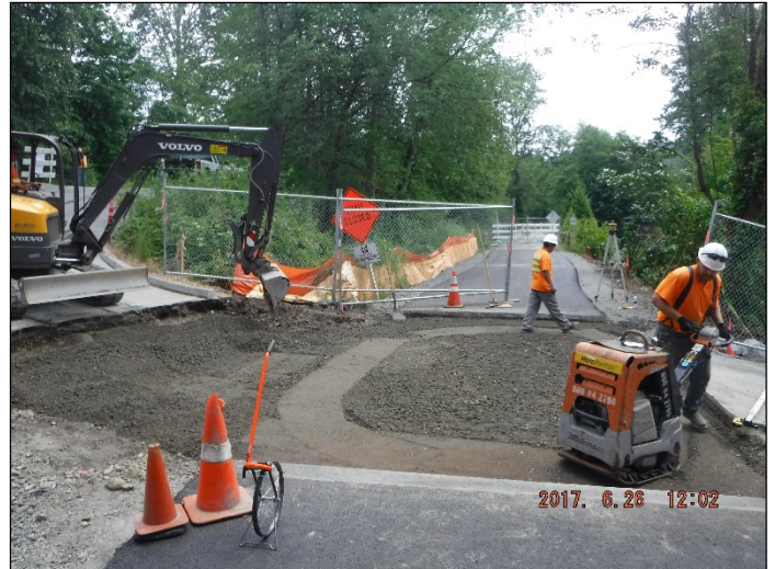
Crushed Surfacing Base Course placed and compacted prior to concrete installation
