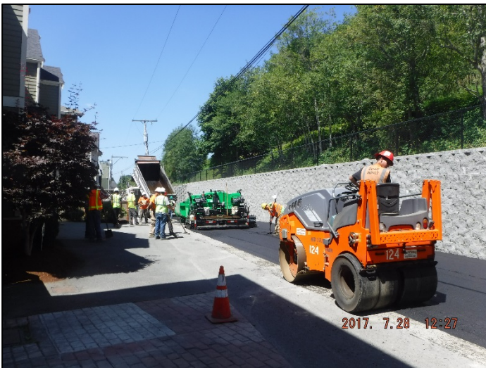
Asphalt paving of Shore Lane between driveways 2 and 3
