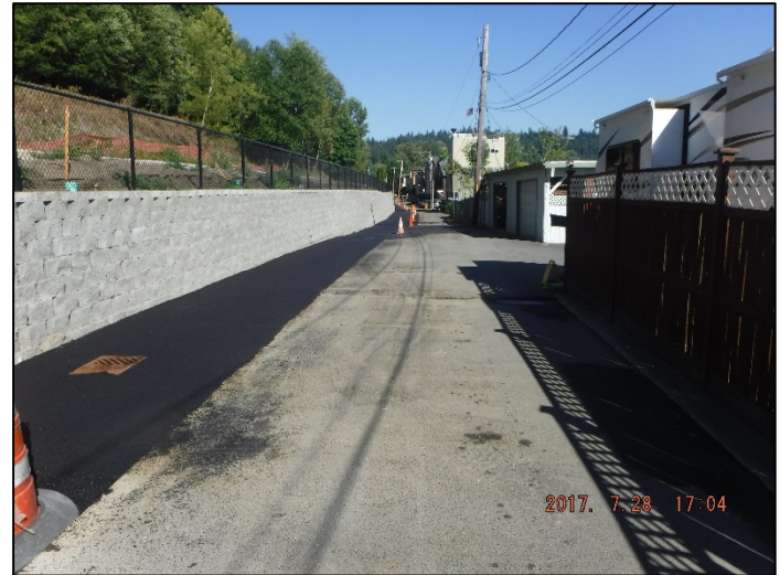
Completed asphalt paving of Shore Lane
