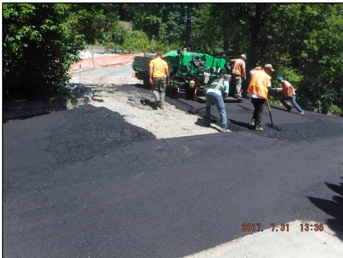
Asphalt installation at driveway 1 approach
