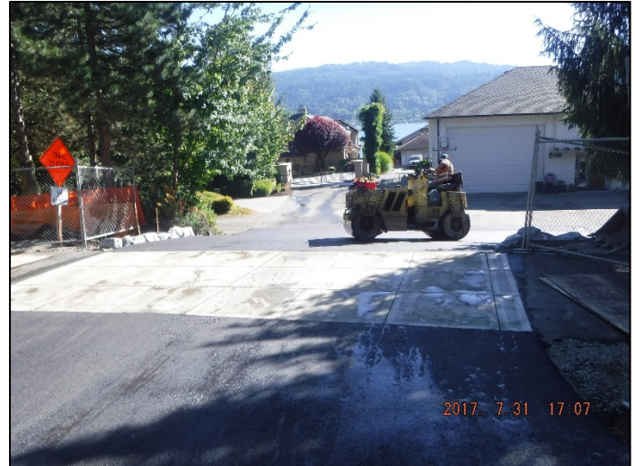
Compacting asphalt at driveway 6 approach
