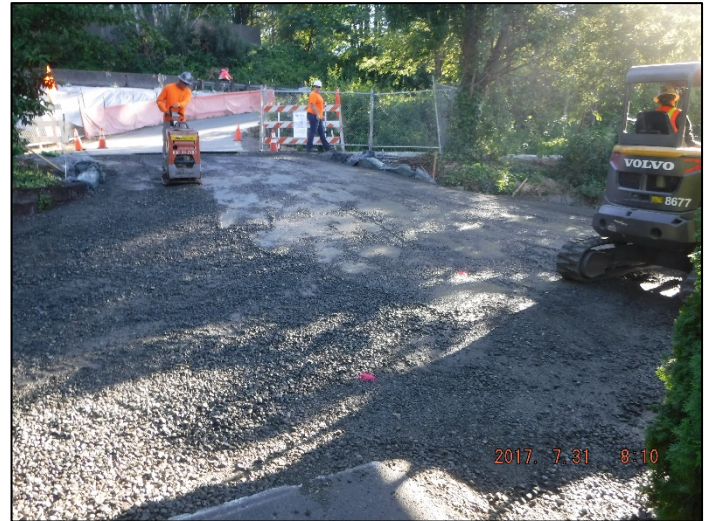
Contractor preparing for asphalt placement at driveway #1 approach
