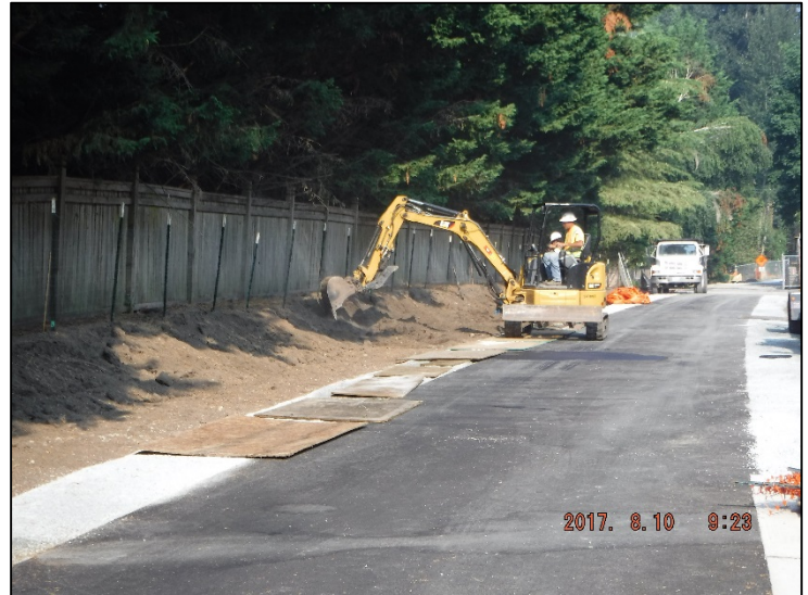
Placing topsoil and preparing planting areas
