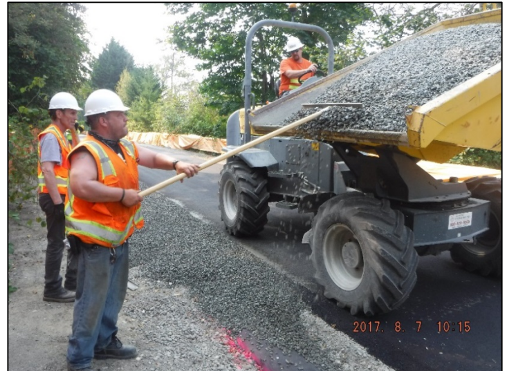
Placing and compacting shoulder rock
