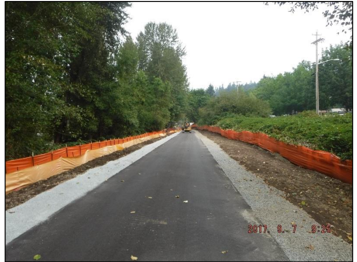
Continued installation of wood chip mulch
