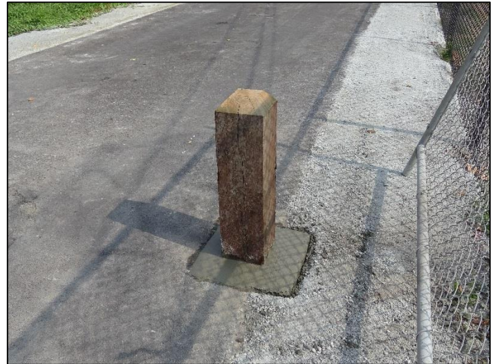
Fixed bollard installation at driveway #2
