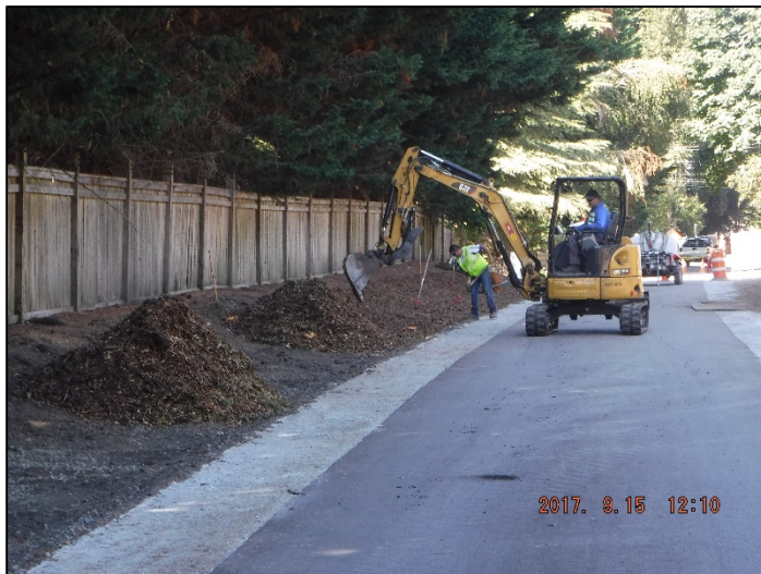
Continued installation of wood chip mulch in preparation of planting.
