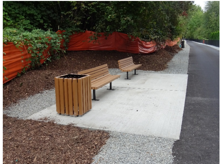
Completed rest area and wood chip mulch installation ready for planting!
