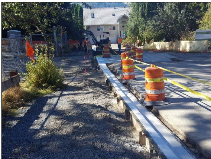
Curb and gutter completion at driveway #7.
