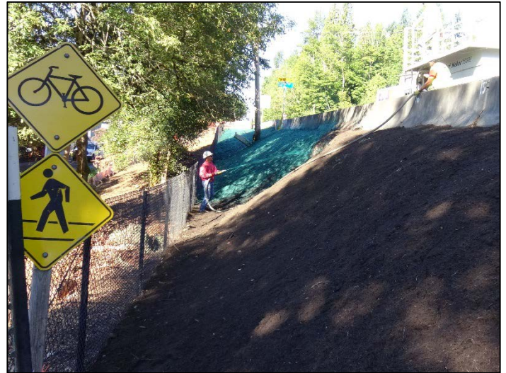
Hydroseed installation on the slope above mitigation site E1
