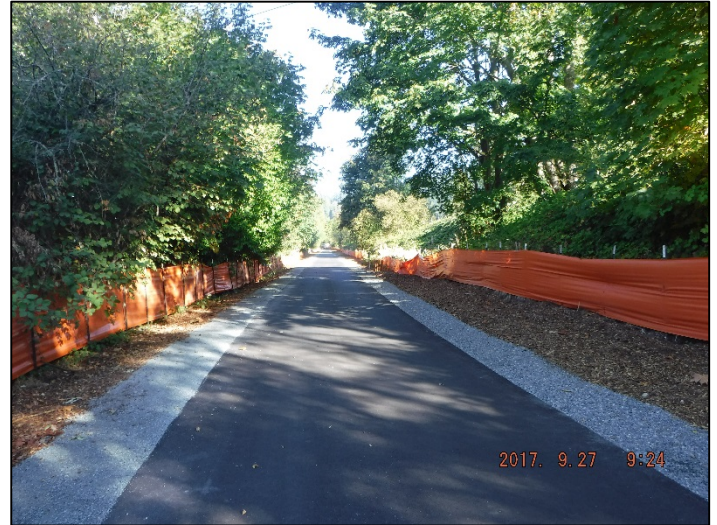
Completed preparation work for landscaping alongside the trail shoulder
