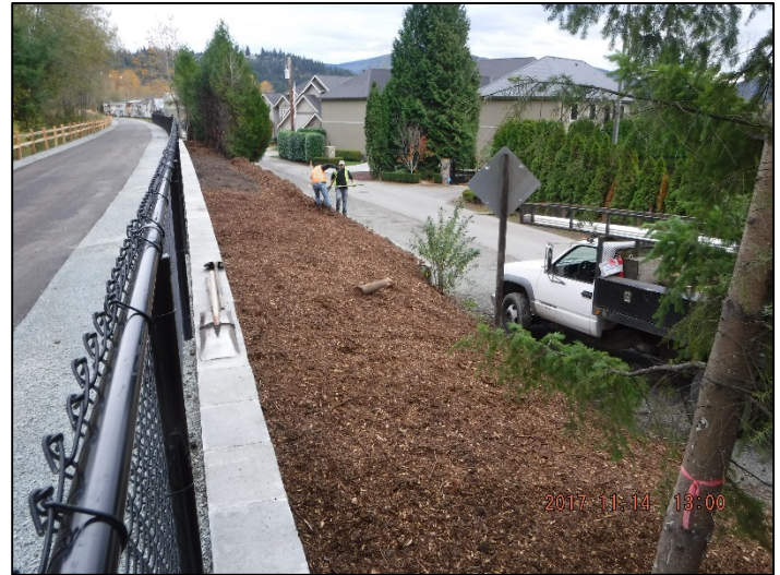
Installation of wood chip mulch in landscaping areas
