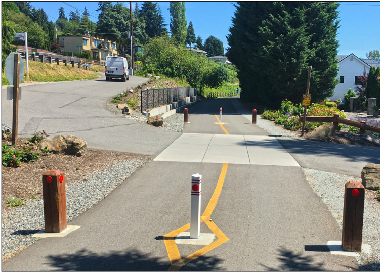
24 intersections on the 3.6-mile South Sammamish B segment will be enhanced with textured concrete, improved sightlines, bollards, striping, consistent signage, and warning bands.
